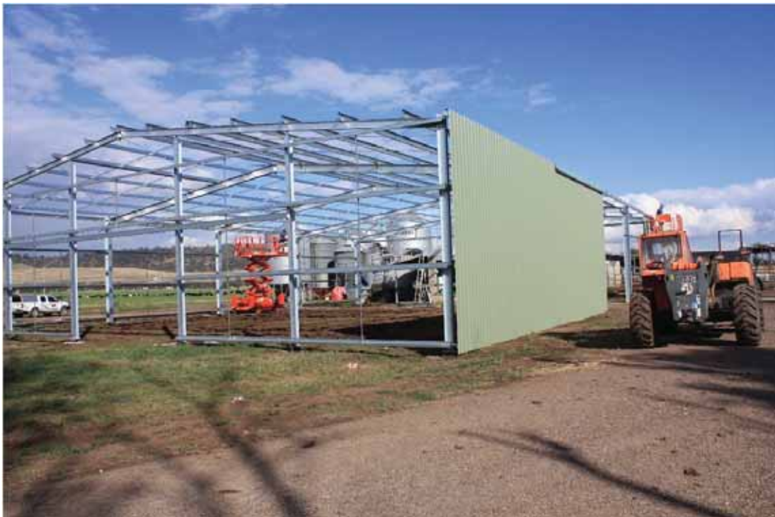
Plate 10 Garoka Dairy Upgrade Works in 2017
