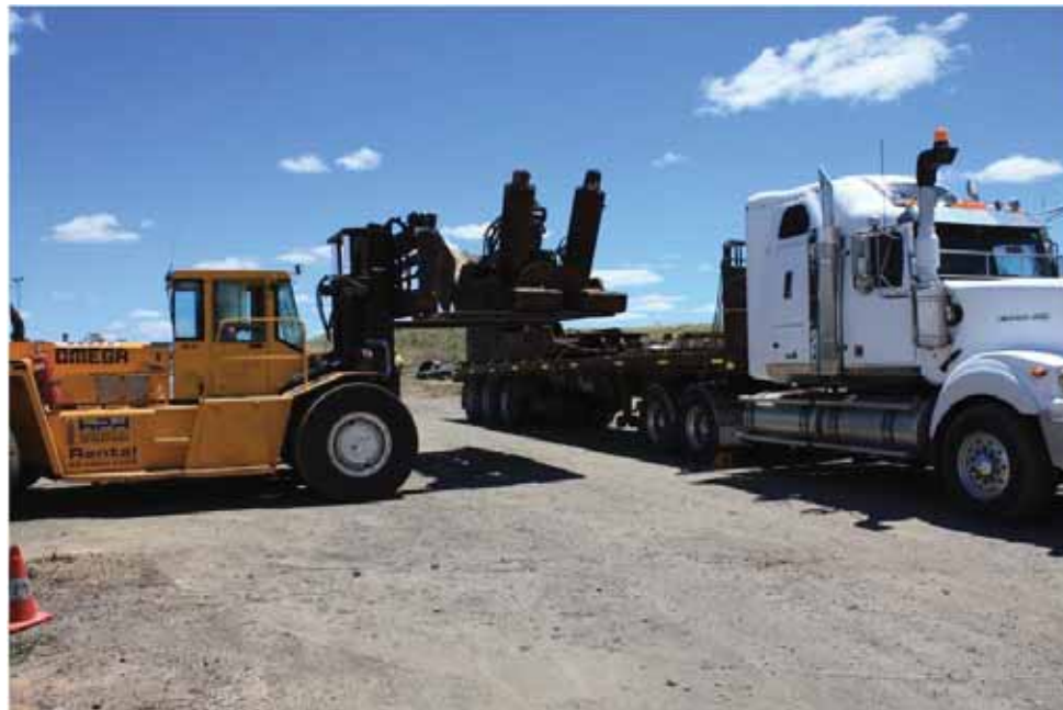
Plate 2 Removal of scrap steel from site 2017
