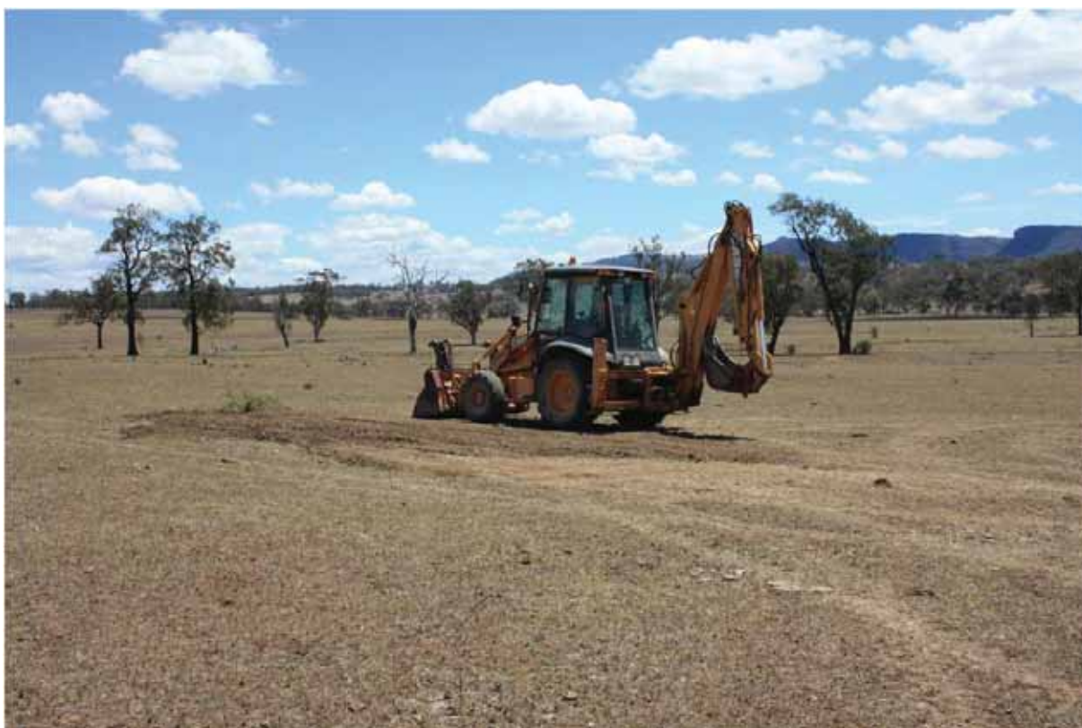
Plate 1 Soil Test Pit Excavation 2017
