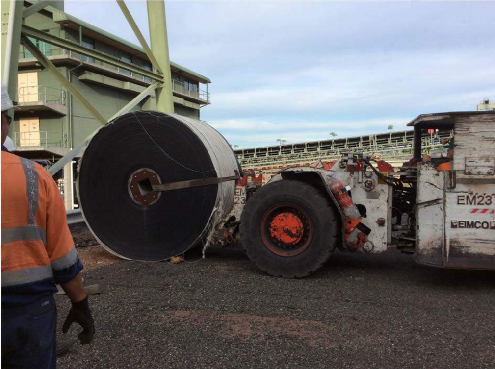
Photo 7 Removal of excess conveyor belt from site
