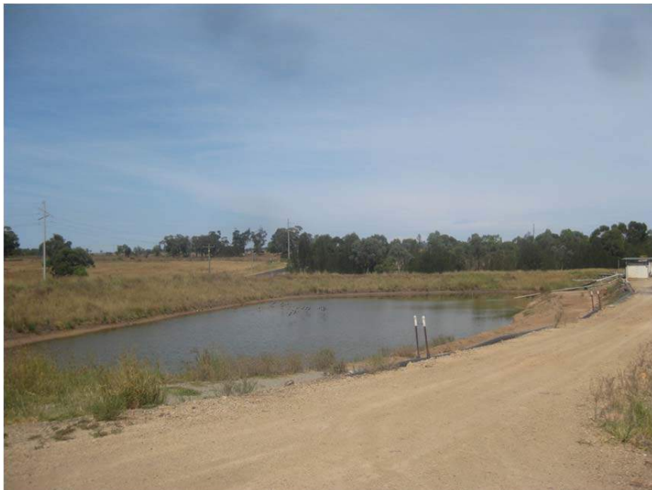
Photo 6 Western Holding Dam,
