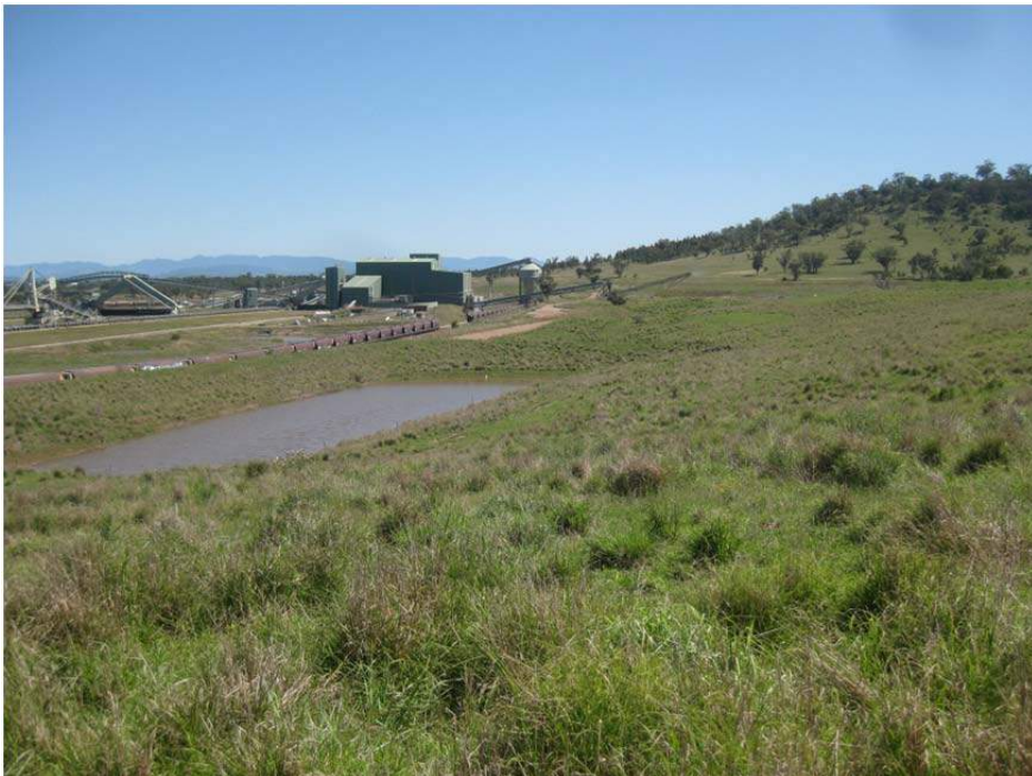
Photo 9 REA Rehabilitation 2015 – western slope looking north
