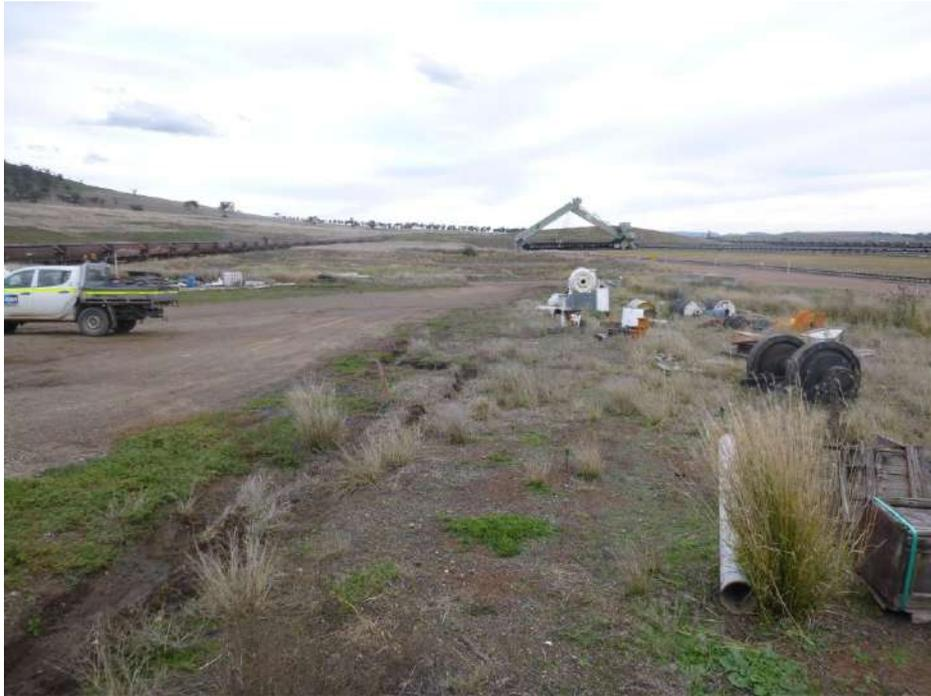
**Photo 7** Minor shaping of drainage line required to direct water to sediment dam.
