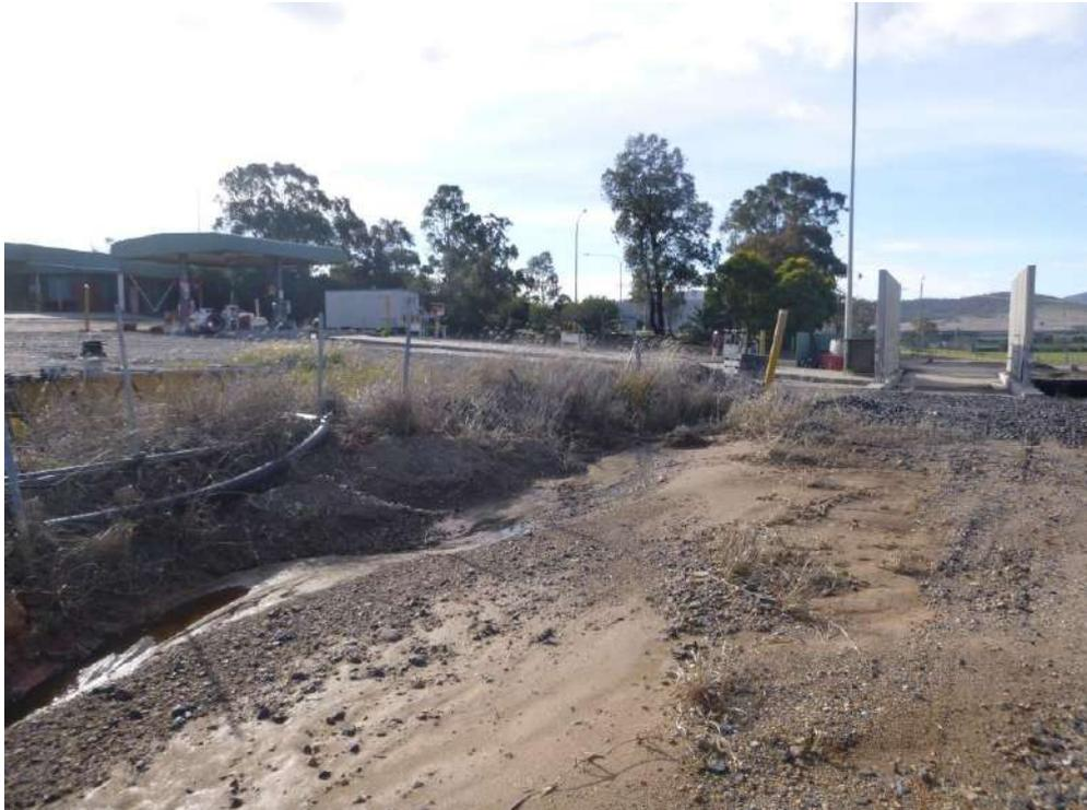
**Photo 16** Sedimentation in Drains around Pit Top to be Removed
