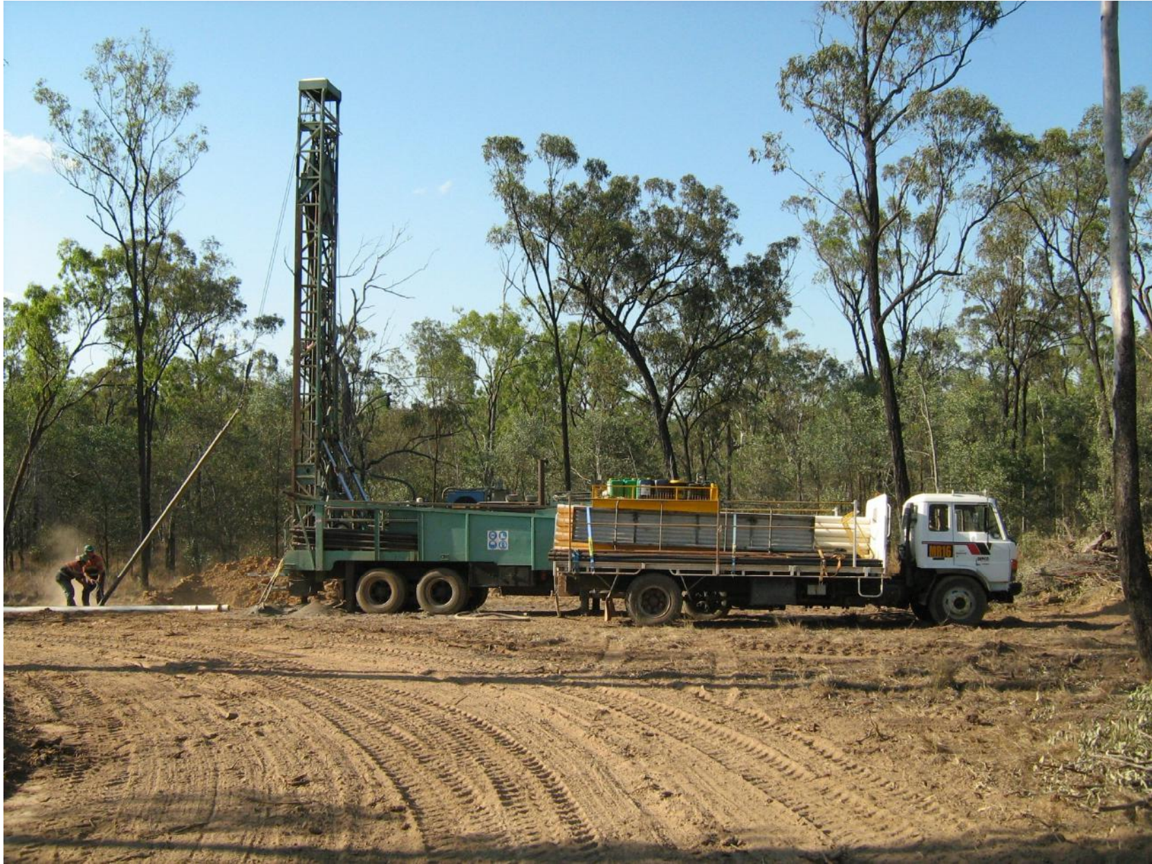
Commencement of Drilling EPC 1548 “West German Creek” 25 October 2011
