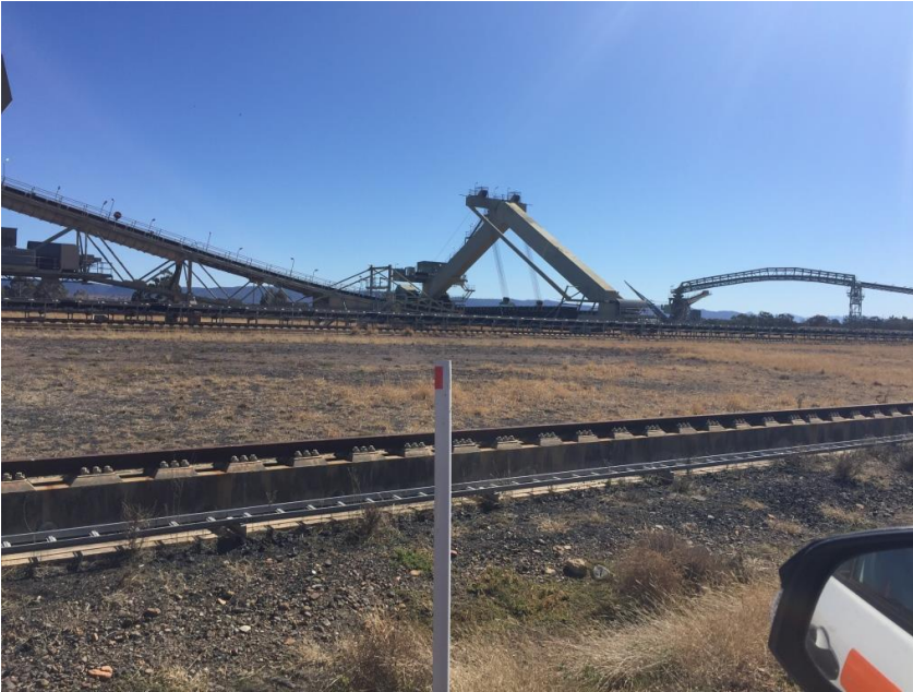
Photo 3 Numerous bare areas at East Site coal stockpiles
