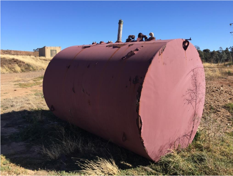
Photo 11 Above ground tank at West Site pit top needs to be moved to a bund or removed from site
