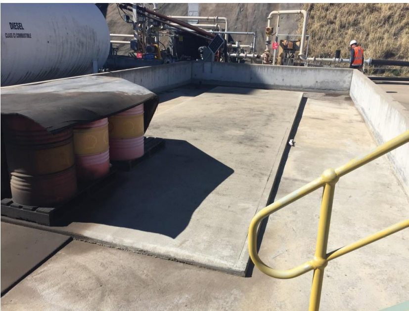
Photo 4 Tanks correctly stored within bunds
