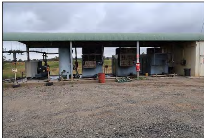
Figure 17 – Air Compressors
