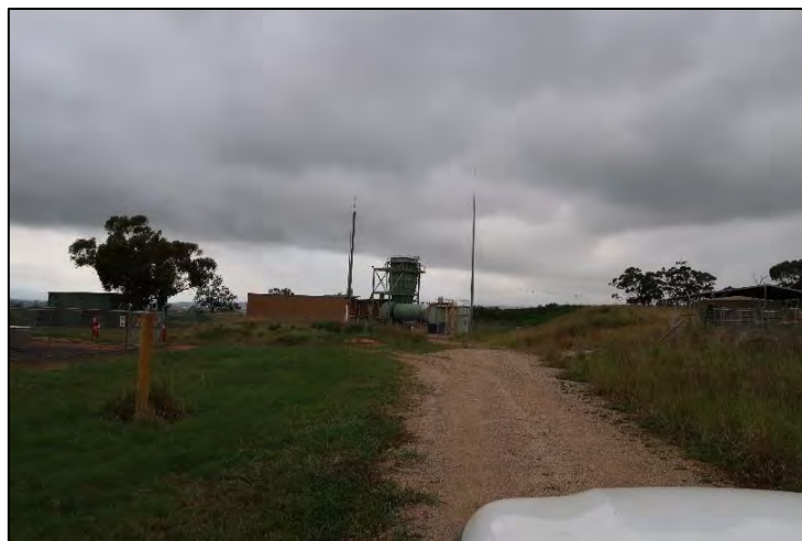
Figure 16 – No. 1 Shaft and Ventilation Fan
