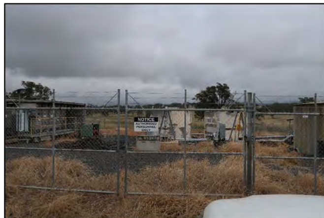
Figure 20 – Pleuger Goaf Dewatering Station
