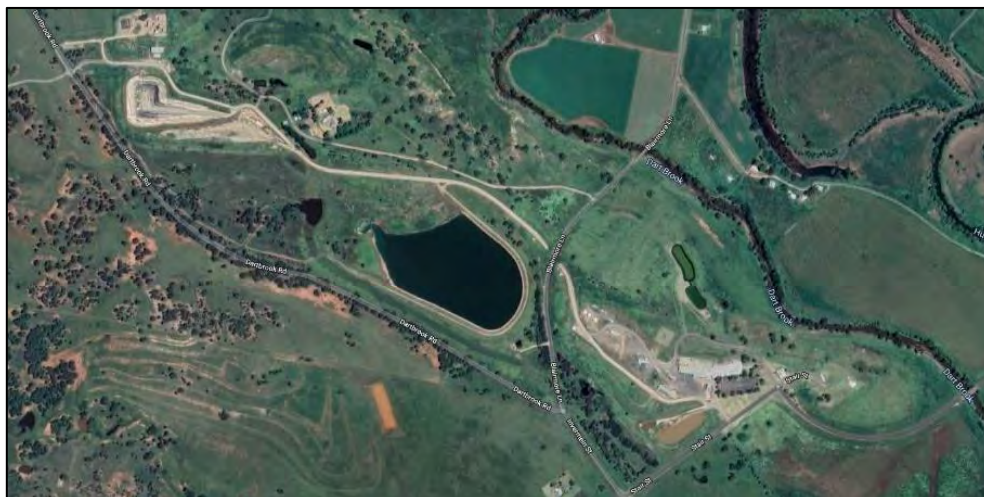
Figure 8 – Wynn and Kayuga Seam Portals – Aerial View
